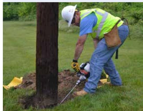
An Osmose contractor bores into a pole to inspect for internal signs of decay.
