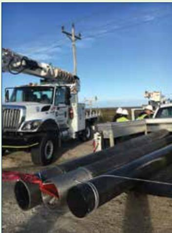
assembly, it can be transported in the back of a pickup truck and hand carried into tight locations. It will not rot, corrode or decay, and is 100% recyclable. Best of all it is rated to withstand winds in excess of 180 miles per hour. Tideland's engineering team chose to install the pole in an area that is most frequently subjected to straight line winds and ocean overwash.
