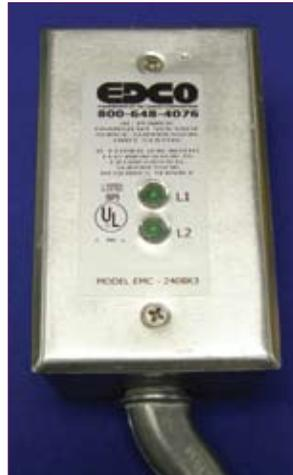
A surge arrester at the meter base offers important protection in lightning prone eastern NC
