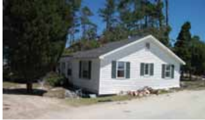
This home was swept into the right of way with the homeowner "aboard."
