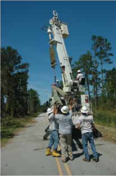
Crews from sister co-ops work to restore power in Lowland. (Carolina Country staff photo)
