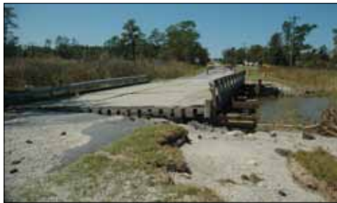
Irene washed out this bridge leading to the Beaufort County community of Hickory Point. (Carolina Country staff photo)
