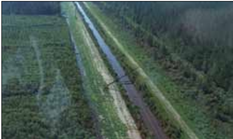
An aerial survey of Hyde County reveals a downed transmission pole. It was built to withstand 130 mph winds. (R. Rouse)
