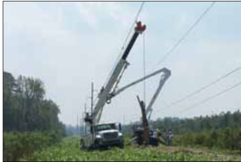
Crews work to replace the Hyde County transmission pole. (Robbie Rouse photo)
