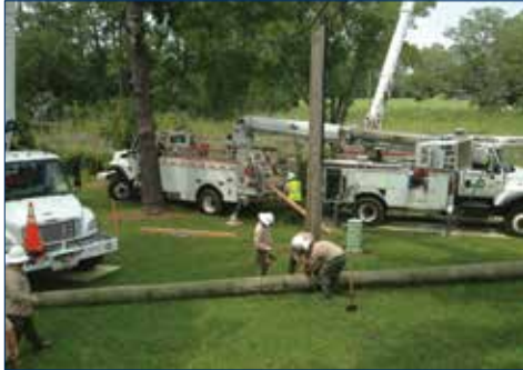
Pee Dee EMC crews work to restore power at Bell Point Road • TW Allen photo
